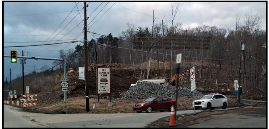
Construction of the SR 611/SR 715 Intersection Realignment
