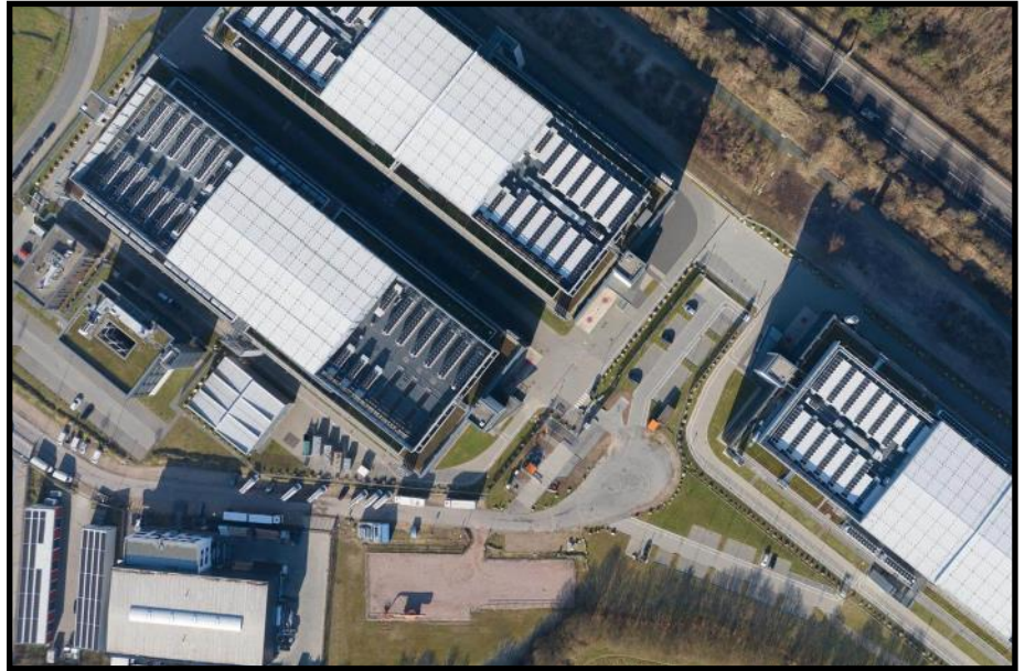
Aerial View of a Typical Data Center
