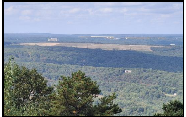
Forest Clearing for the Swiftwater Solar Facility
