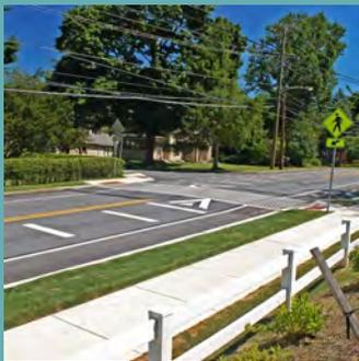
**Description:** Marked and elevated areas that are an extension of the sidewalk at mid-block locations or intersections. They can be used to increase pedestrian safety, calm traffic, and add to the community character. When used for traffic calming, they are most effective when placed in series. They may be constructed of asphalt, brick, or stone pavers.
