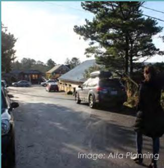
**Description:** A narrow roadway without pavement markings that is intended to support walking, biking, and driving in the low-speed travel way. These roads serve bi-directional traffic with no pavement markings, but their narrow design encourages lower speeds.
