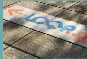
**Description:** Wayfinding markings that are placed on the pavement to identify a facility and provide basic information, such as directional arrows or mileage.
