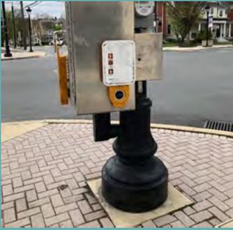
**Description:** Traffic signal equipment for pedestrians can include pedestrian pushbuttons, accessible pedestrian signals, passive detection for bicyclists or pedestrians, pedestrian signal heads, and pedestrian countdown signal heads. Accessible pedestrian signals (APS) communicate information about the WALK and DON'T WALK intervals for pedestrians who are blind or have low vision. Countdown pedestrian signal heads show how much time remains before the traffic signal changes.
