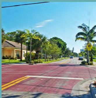
**Description:** An entire intersection, including crosswalks, that is built level with the sidewalk and/or has textured pavement. Similar to a speed hump or table, a raised intersection provides a vertical deflection to slow traffic. The elevated crosswalks also make it easier for pedestrians to cross the street. Raised intersections can be built with a variety of materials, including asphalt, concrete, or pavers.
