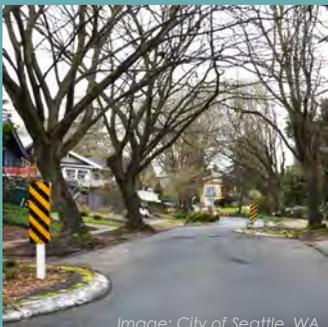
**Description:** Series of three bulb-outs, staggered at mid-block locations on alternating sides of the street. Chicanes force drivers to slow down to negotiate through the series of extensions. Chicanes can include landscaping to improve the street appearance, but will reduce on-street parking.
