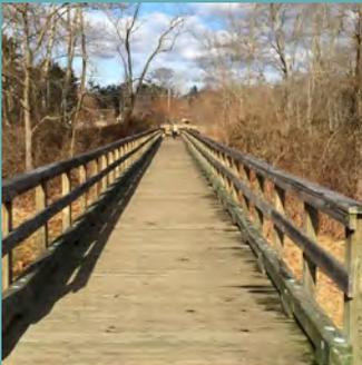
**Description:** Elevated walkway that is constructed as a series of low-height bridges through sensitive areas with seasonably variable water depths or low strength soils, such as wetlands. Boardwalks typically include a curb or handrail along at least one, often both, edges.
