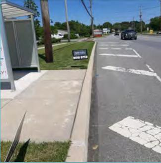
**Description:** A level loading area where the front, side, or rear door of a bus open to receive and discharge passengers. The clear area allows deployment of a front door ramp on the bus. The loading pad should be a firm and slip-resistant surface, such as concrete. Additionally, it should be free of conflicts, such as landscaping or street furniture. The loading pad should be a minimum of 5 feet wide along the curb and 8 feet deep.
