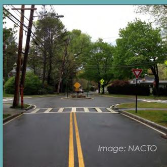
**Description:** A roundabout with a small diameter and traversable central island. Mini-roundabouts offer benefits similar to roundabouts, but with a smaller footprint and less cost. Mini-roundabouts are typically used in urban or small town settings on roadways with low speeds.
