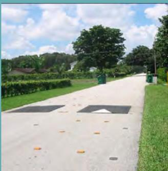
**Description:** Speed humps or speed tables that include wheel cutouts to allow larger vehicles to travel without slowing down to travel over the hump. They are intended to allow emergency vehicles or transit vehicles to travel unimpeded.
