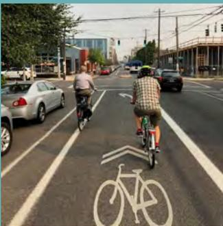
**Description:** A roadway with signage and pavement markings to indicate the use of a travel lane by both bicycles and motor vehicles. Pavement markings may include a “sharrow,” which is a bicycle symbol with two chevron arrows denoting the direction of travel.
