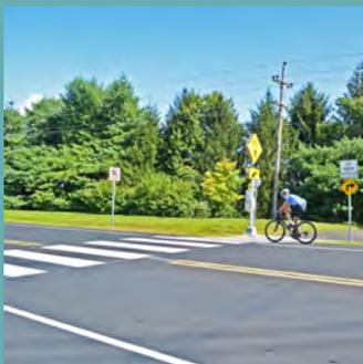
**Description:** A crosswalk that is not located at an intersection. Additional warning devices for drivers are required to increase pedestrian safety compared to typical crosswalks at intersections. A mid-block crosswalk can include advance signage and pavement markings. Other design treatments could include a pedestrian refuge island or raised crosswalk.
