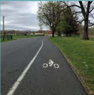
**Description:** A portion of the roadway that has been designated by striping, signage, and pavement markings for the preferential or exclusive public use by bicyclists. Bicycle lanes are located directly adjacent to motor vehicle travel lanes and operate in the same direction as motor vehicle traffic.
