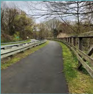
**Description:** A combined bikeway and walkway that is designed for shared use by bicyclists and pedestrians of all abilities, as well as other non-motorized modes of transportation. Trails along or adjacent to a roadway are physically separated from vehicular traffic by a verge, fencing, or other barrier.
