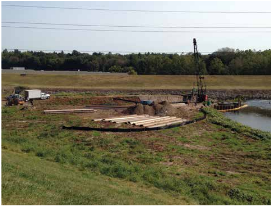
Expansion construction of the Stroudsburg Waste Water Treatment Plant
